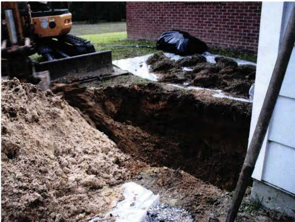
Picture 2: UST 546LaurelBB excavation in progress.
